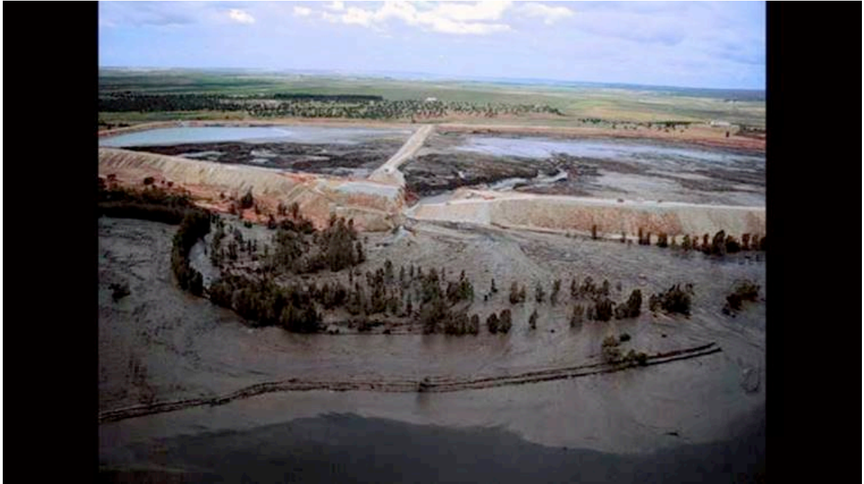
A breached (lead/zinc) earthen dam in Spain. The culprit in this instance was Boliden, a Canadian mining company. (April 25, 1998)
